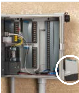
WIFIKIT Wi-Fi accessory for ICC2 Controllers, managed by Centralus Software page 108
